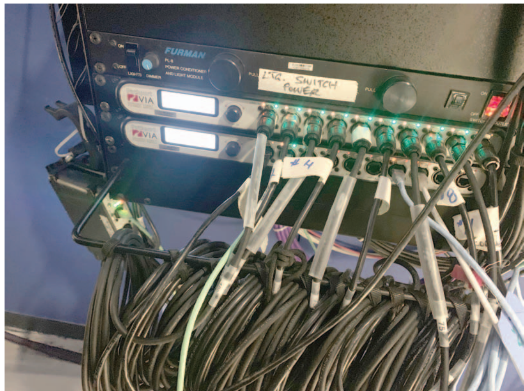
Pathway Connectivity VIA Ethernet switches in The National news studio at the CBC.
