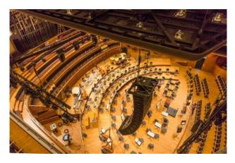
Part of the lighting park has been installed on eight, electromechanically driven, light bridges. In the Main Hall, the lighting equipment has been installed also under the balconies surrounding the hall. P.S. TEATR fitted the National Music Forum with altogether: around 520 pcs of luminaires and floodlights and 116 pcs of moving heads type devices.
