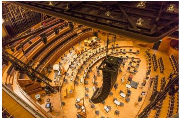
Part of the lighting park has been installed on eight, electromechanically driven, light bridges. In the Main Hall, the lighting equipment has been installed also under the balconies surrounding the hall. P.S. TEATR fitted the National Music Forum with altogether: around 520 pcs of luminaires and floodlights and 116 pcs of moving heads type devices.
