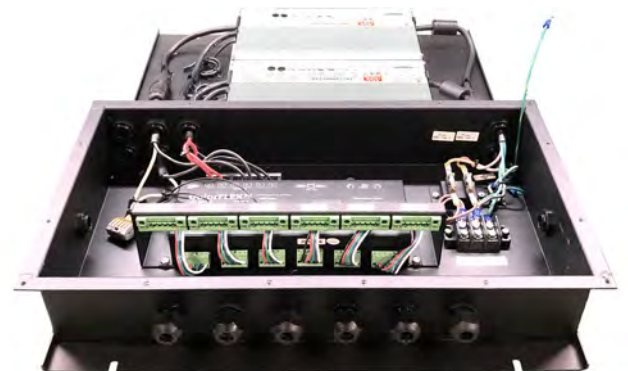
Custom low voltage QolorFLEX Dimmer boxes
