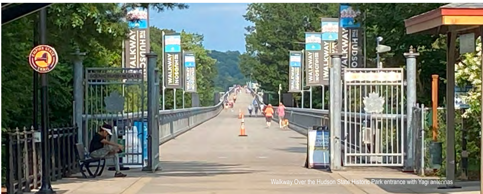
Custom stainless steel enclosures shown on the bridge
