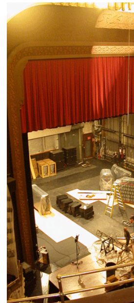
Cutting a hole in the proscenium cluster
