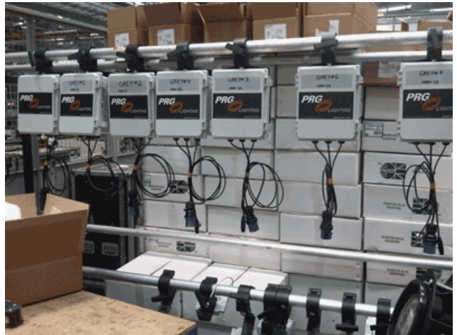
Directional antennas on focusable brackets
