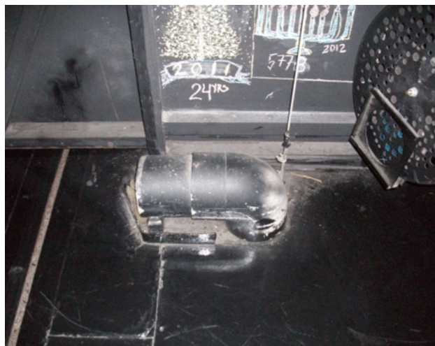
Fog vent in the stage door
